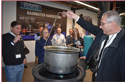
Local 130 Apprenticeship Training Director Jim Majerowicz shows members of the tour one of the filters of the rainwater harvesting system.
