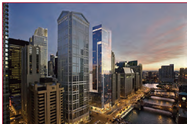
OneEleven West Wacker Tower → 111 West Wacker Drive, Chicago Owner: Related Midwest General Contractor: Lend Lease (US) Construction, Inc.
