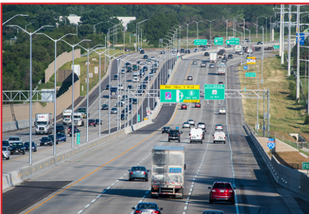
Jane Addams Tollway (I-90) Reconstruction
